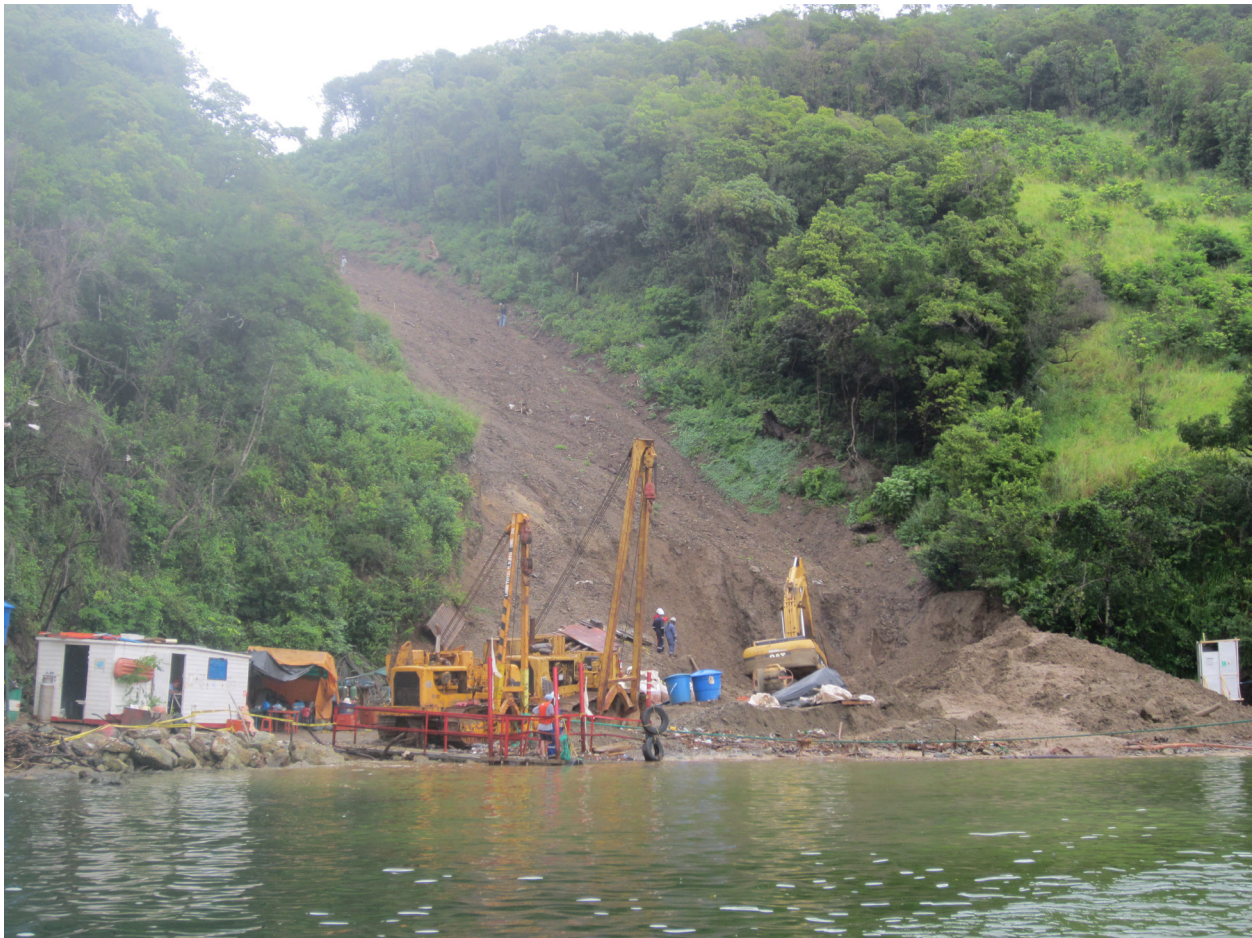
Photo 1. Beginning of the deforestation and construction of the gas pipe at Obispo Isthmus in the year 2014. Photographed by Luis Cova.
